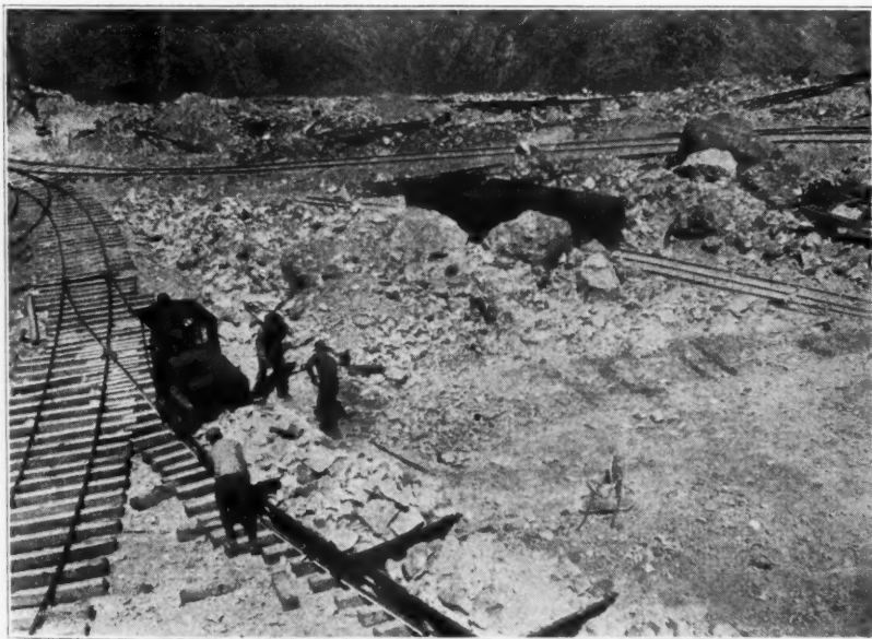
The Quarry Floor and Tracks
